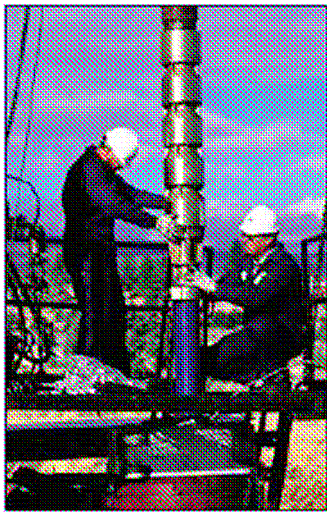
Figure 35: Technicians installing a vertical turbine pump—for a description of the pump, see the chapter entitled Drilling Technologies
