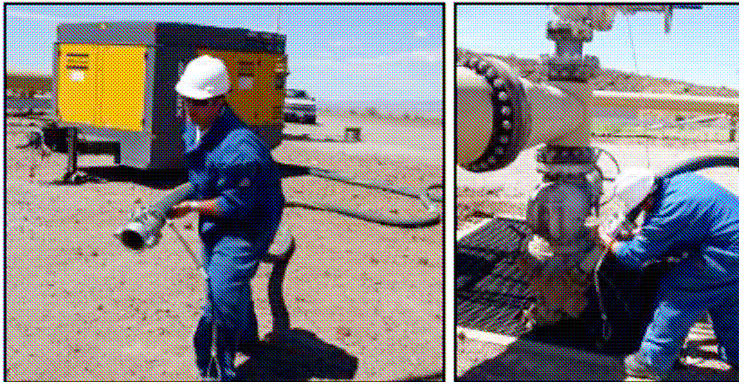
Figure 31: Technician inducing well flow using airlift method
