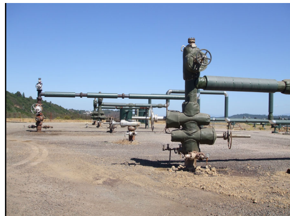
Figure 15: Drill pad with multiple wellheads
