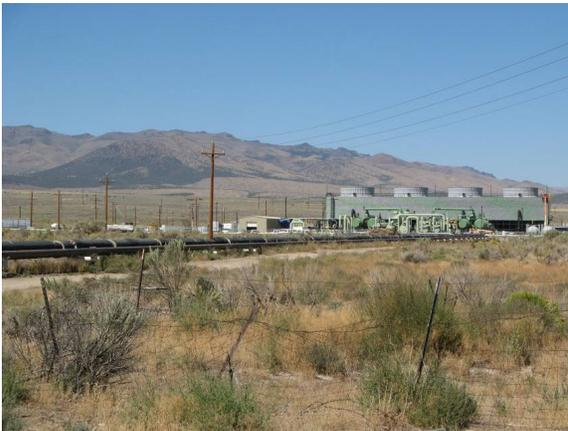
While today water cooling is mostly used in higher-temperature non-binary facilities due to the use of the geothermal fluid for cooling, a few existing and developing binary facilities in the U.S. utilize water-cooled systems. The binary plants at Heber, East Mesa and Wendel-Amedee, all in California, use water cooling. The Raft River geothermal plant, the first in Idaho, is a binary facility that uses water cooling.
