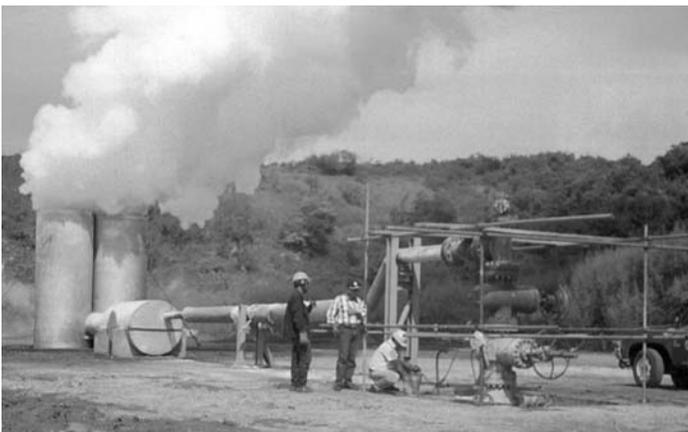
*Momotombo well OM-53. Production testing and gas sampling.*
