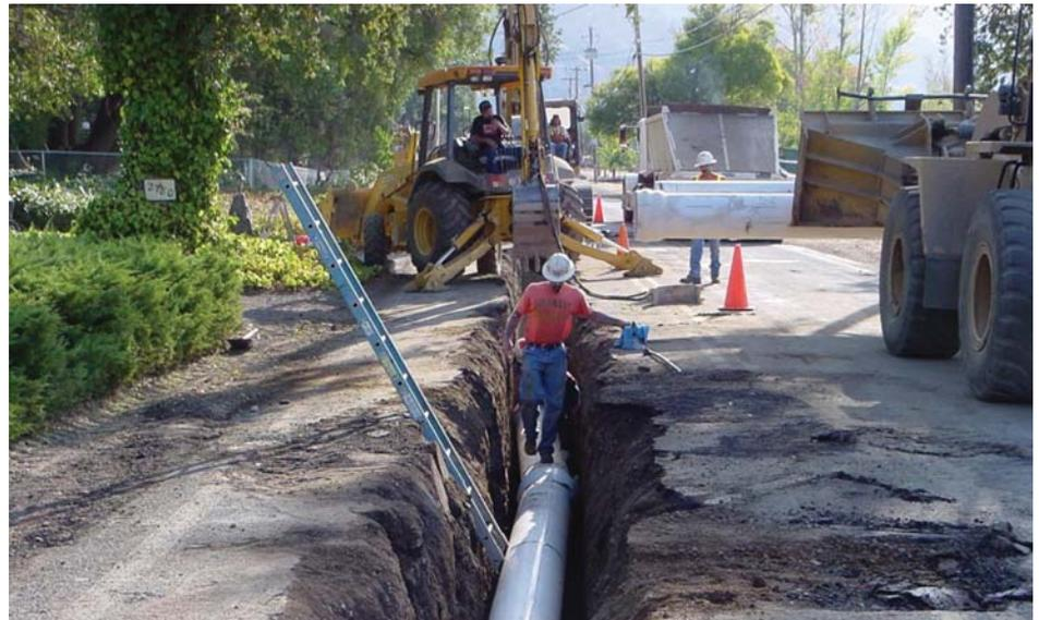
*Lake County effluent pipeline construction used existing rights-of-way wherever possible to minimize environmental disturbance. Pipeline diameters ranged from 16 to 20 inches, using PVC, welded steel, and ductile iron pipe.*
