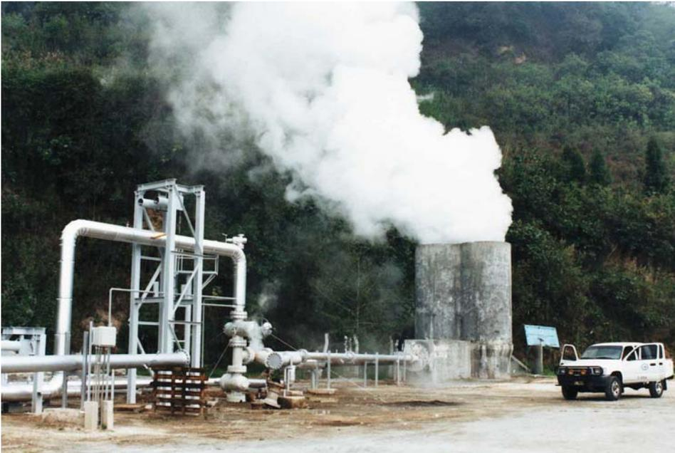
*Well at ZCQ-6 at Zunil-I during production test. The 1143 m deep well was completed in 1981 and side-tracked in 2001.*
