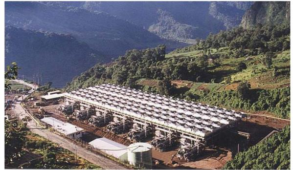
*The 28.6 MW gross (24.6 MW net) binary geothermal power plant at Zunil-1 that went into commercial operation in 1999. It consists of seven identical air-cooled OEC Modules (photo courtesy of ORMAT International, Inc.)*
