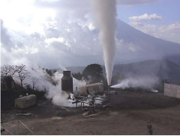
Initial discharge of well AMJ-2 (AMF-6J in INDE's nomenclature) at Amatitlán; Volcán de Agua is in the background. The 1,700 m deep well was completed in August 2000. It was drilled with funds from a JICA grant.
