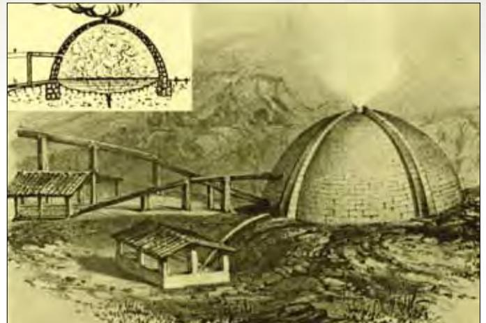
A *lagone coperto* ("covered pool"), shown above, is made out of bricks. It collects steam and boron-bearing waters from geothermal pools in the Southern Tuscan Hills. Note the pipes for extracting the steam (a) and boron-bearing geothermal waters (b). The waters, piped into nearby tanks heated by the steam, will evaporate—leaving the borax. COURTESY OF ENEL.
