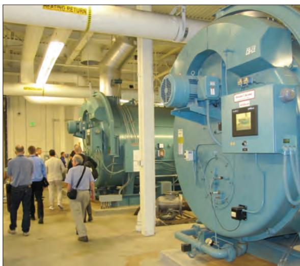
New sources of geothermal heat allowed the Peppermill to retire its Cleaver Brook natural gas boilers in 2009.
